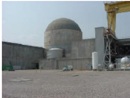
*The dome-shaped containment building at the Shearon Harris Nuclear Power Plant near Raleigh, NC*
